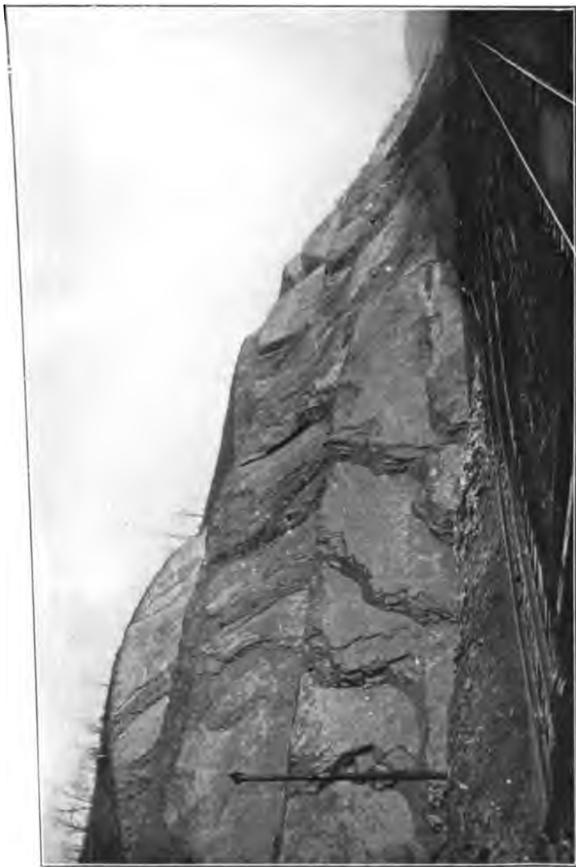
PLATE XXXVII.—View showing Flaggy Character of Catskill Sandstone in Doe Gully Cut of Baltimore and Ohio Railroad.
